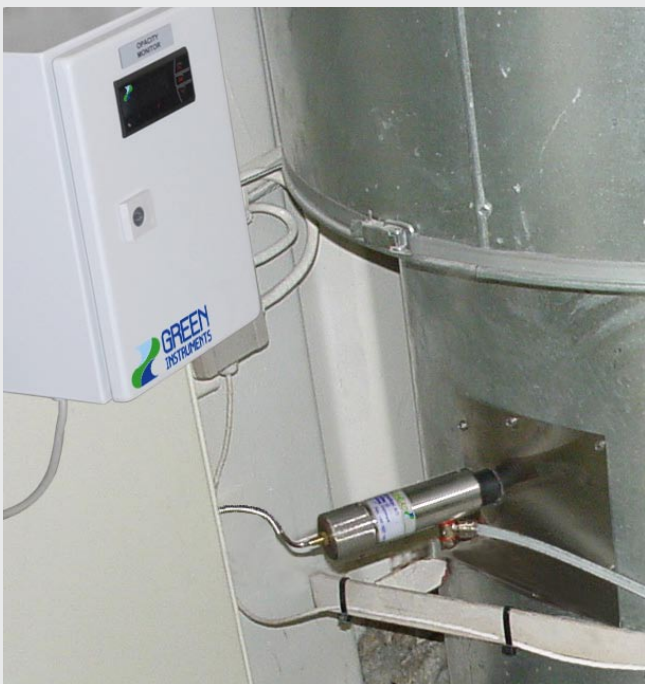
An installation of a G1000 Smoke Density Monitor with the monitoring unit and one optic head
