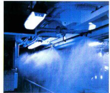
Machinery spaces and local protection
